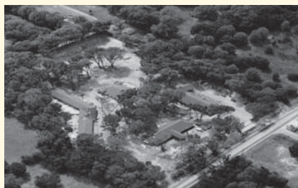
Construction begins in early 2000
